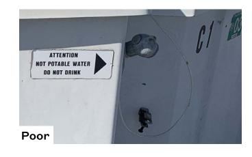
Check that the rinse hose is available and can be used to clear out lingering sewage from the inside of the dump station after boaters are finished
