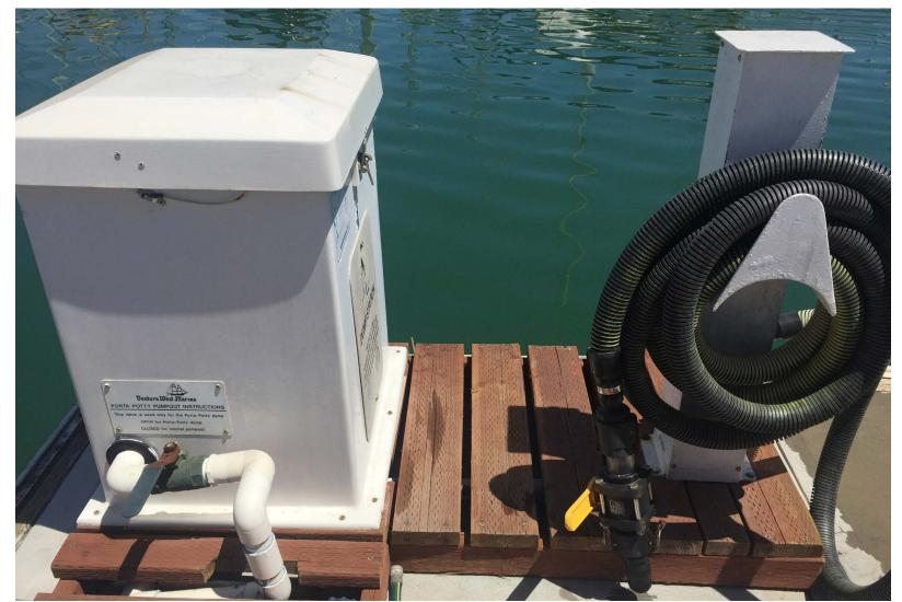
Motorized dump station requiring the manual opening of its ball valve for drainage Photo by TBF
