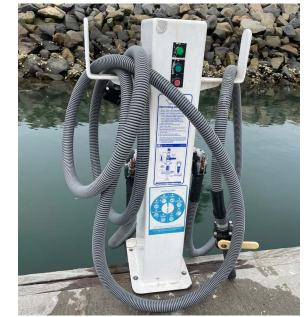
Pumpout unit retrofitted with a port-a-potty wand attachment Photo by TBF
