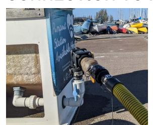
A gravity-drained dump station manually connected to a pumpout unit's infrastructure by attaching the pumpout waste fitting Photo by SFEP
