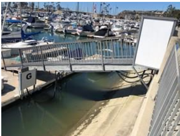
View of subject's walkway to boat slip area.
