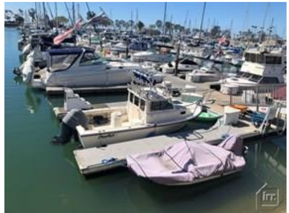
View of boat slips, showing signs of deferred maintenance.
