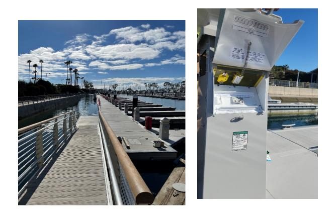
Power pedestals serve as multi-purpose devices, which supply power, water, internet, ground fault protection, remote metering and lighting to boats of any size and magnitude. Many boats require shore power to run onboard lighting, air conditioning, pumps, and small appliances while the vessel is docked. Power pedestals provide all of these essential utilities and capabilities within a single unit.
