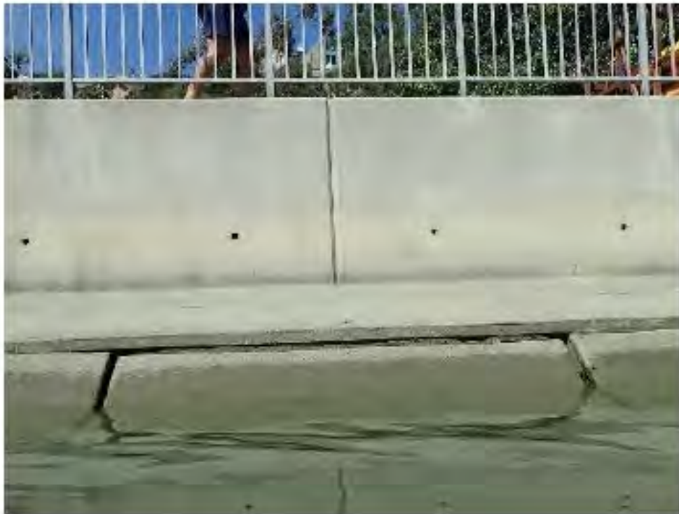
California Coastal Commission 5-19-0971 Exhibit 10 – Seawall/Revetment Repairs (Repair Type 2) Page 2 of 3
