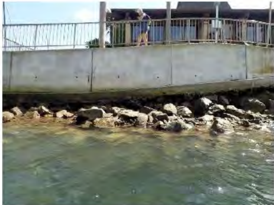
California Coastal Commission 5-19-0971 Exhibit 10 – Seawall/Revetment Repairs (Repair Type 3) Page 3 of 3
