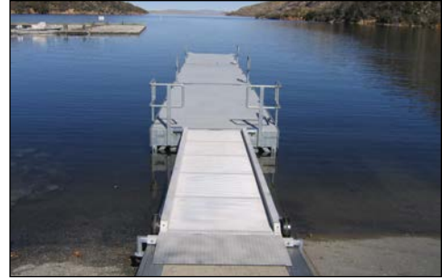
dubbed 2008 dual-rail guided boarding float
