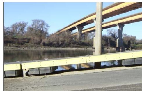
30 inch max. boarding float height
