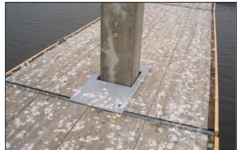
sliding pile yoke cover on square pile
