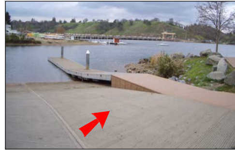
launching ramp apron merging with vertical curve
