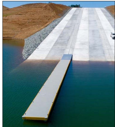
cable-guided boarding float
