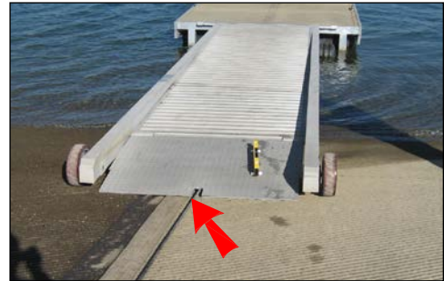
gangplank with centerline cable
