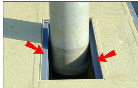
pile yoke rub strips
