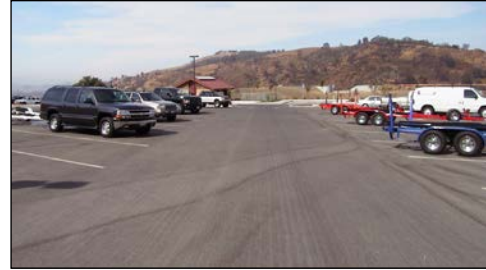
large visual expanse of AC paving
