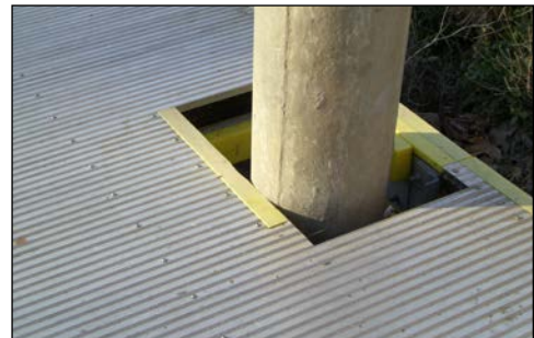
interior pile yoke flush with deck
