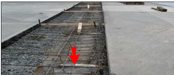
closure section under construction
