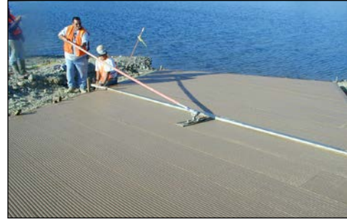
creating diagonal V-grooves in wet concrete
