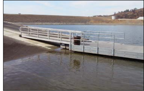
gangplank access to boarding floats
