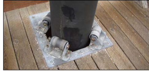
pile rollers wearing against round pile
