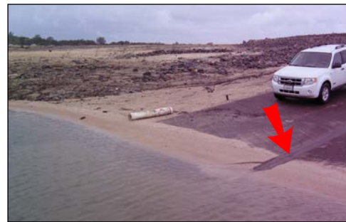
effectiveness of V-grooves in moving silt across and down a ramp
