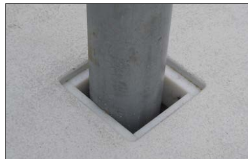
square pile yoke with rub strips
