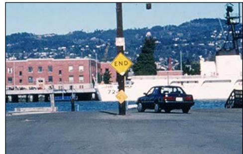
boat launching ramp with safety warning signs: at end of access road, and at top of launching ramp
