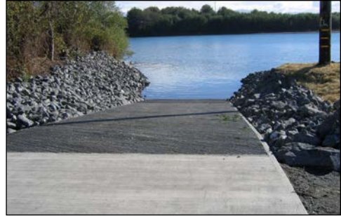
single-lane launching ramp
