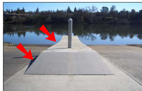
matching width of gangplank and float
