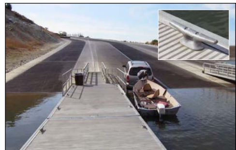
minimum of 5 ft clear between edge hardware
