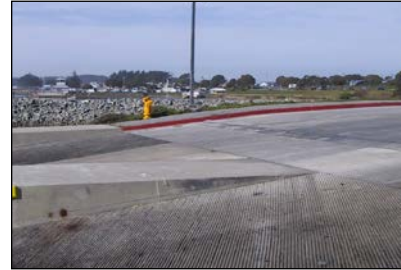
boarding float abutment
