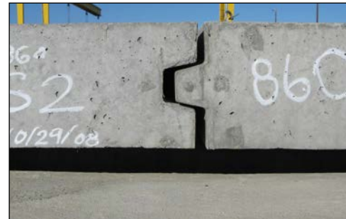
precast concrete panel keys
