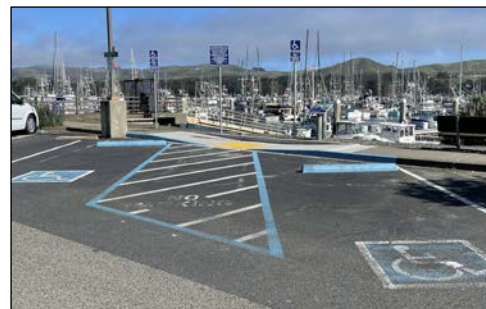
accessible ramp and access aisle
