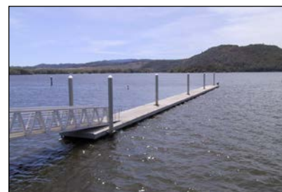
Case #1. gangway and boarding float ARE NOT ON launching ramp
