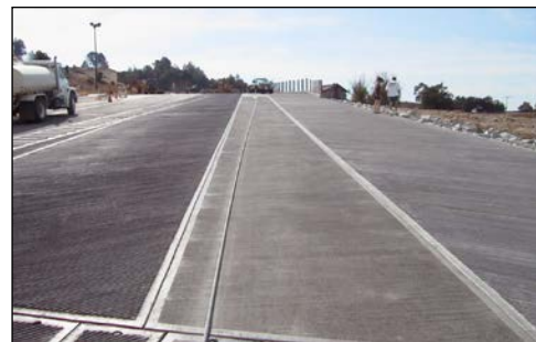
3-inch shiny edges delineate launching lanes and construction joints
