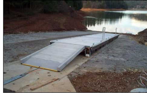
self-adjusting boarding float at rest on launching ramp
