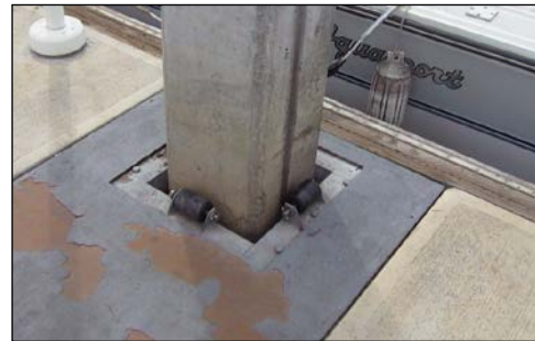
square concrete guide pile
