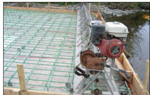
gasoline powered vibratory screed
