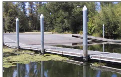
removable exterior pile yokes around steel guide piles
