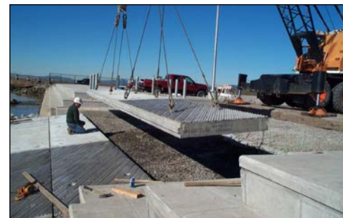
large precast concrete panels being placed
