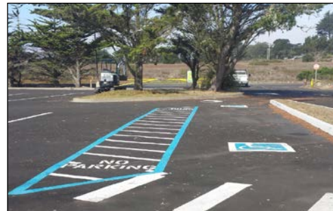
45 degree diagonal lines on 3 ft centers plus "NO PARKING" notification
