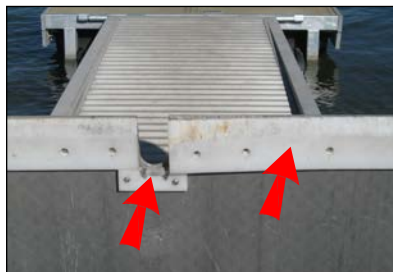
gangplank lifted up to see cable slot and wear slip
