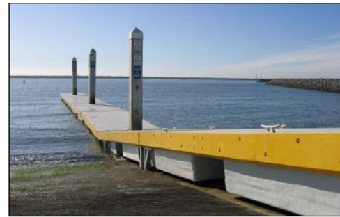
non-articulated float section at far end
