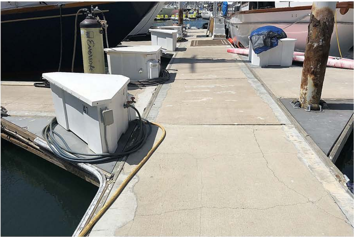
Photo : Piles in a poor condition.
