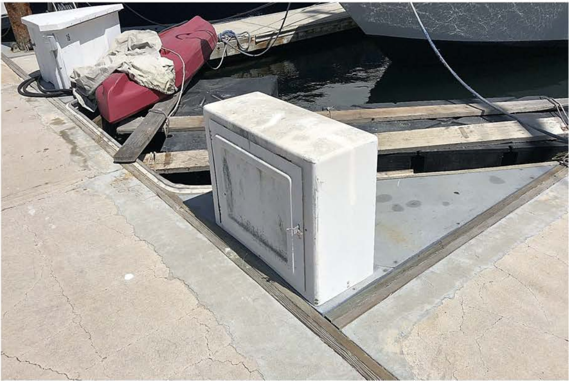
Photo : Repaired finger
